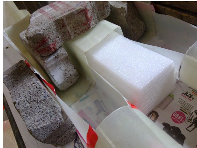
17. Meanwhile the Coke bottle moldings are attached to the jet channels base by taping mylar and glassing. I managed to go from square to round.
