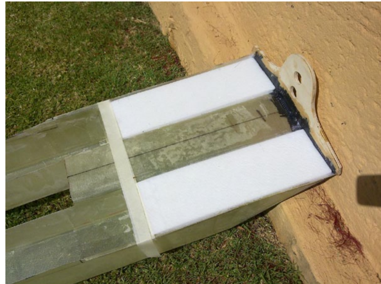
38. The temporary supports are removed and the wing base is made up of a foam sheet and epoxied in.
