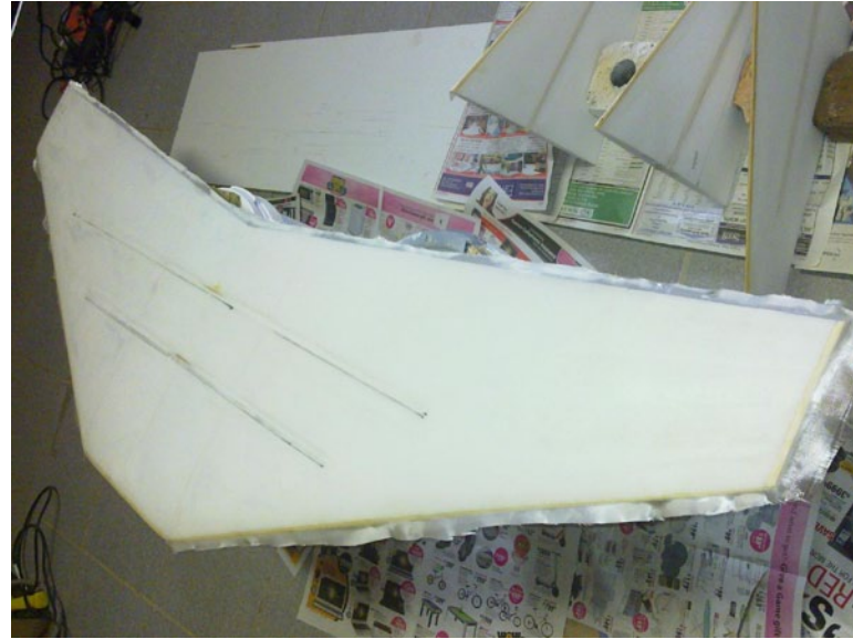
26. The under side blown dust free and cloth resined in place with a little overlap. Old plastic credit card spread epoxy.
