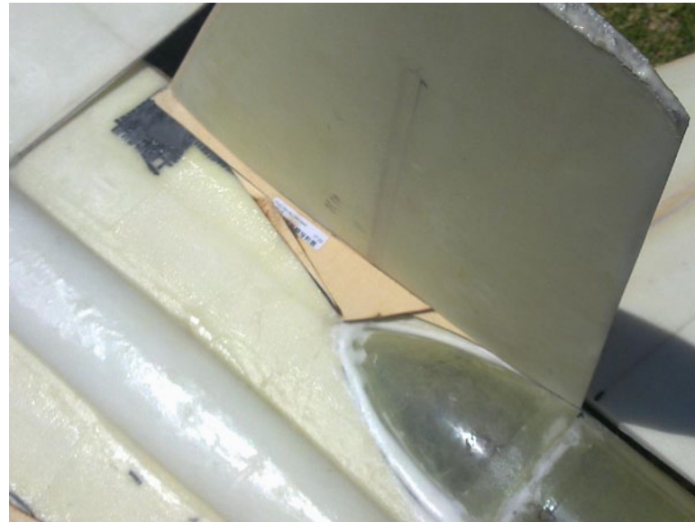
68. I need a third anchor point, so added a plywood foot.
